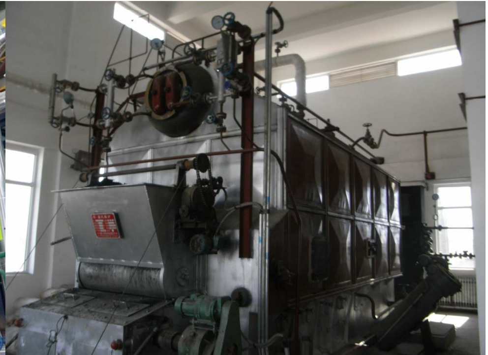
Coal Fired Boiler (2t/h, 3MPa)
